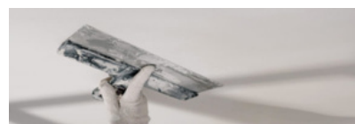
Finished gypsum board
