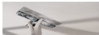
Finished gypsum board
