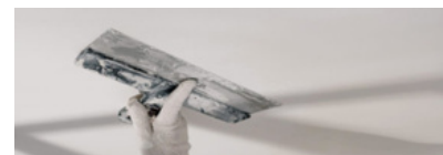
Finished gypsum board
