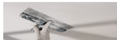
Finished gypsum board
